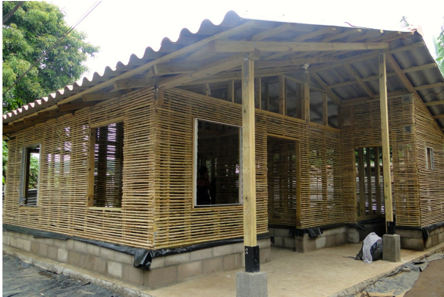
Figure 1. Prototype cane and mortar house under construction (El Salvador Project, 2012)
