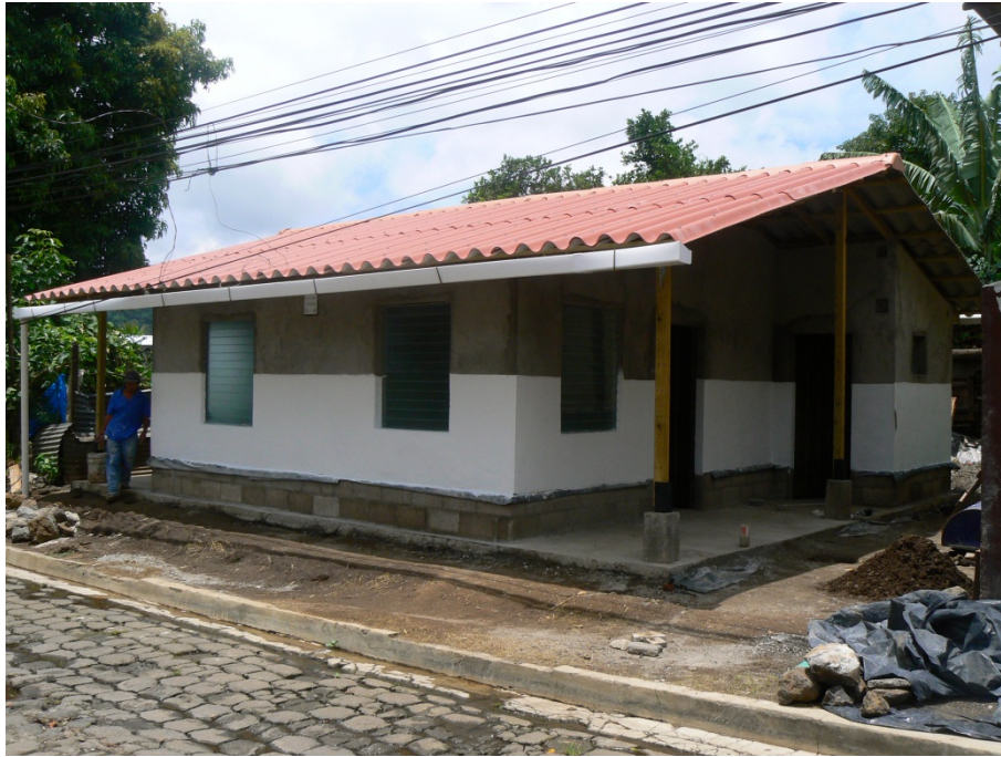
Figure 4. Prototype cane and mortar house, completed in 2012 (El Salvador Project, 2012)
